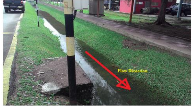
Figure 1: Flow through the Grassed Swale Type B
