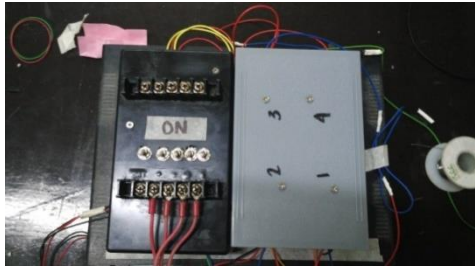
Figure 5: Solar Measurement Device
