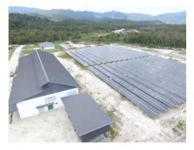
Figure 2: Centralized Solar Hybrid System in Bario [10].
