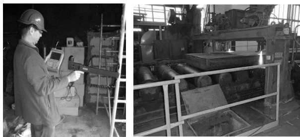
Figure 2: (a) Situation the measurement of interference into electric cable, (b) Situation the measurement of voltage difference grounding pins (c) The measurement processing examples in future server room and industry area placement
